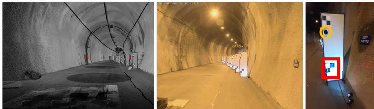
Figure 3: Scene as seen by the sensor system. On the front left the fire cup, on the back right ten laser targets. The detailed view shows the attached black&white targets (red square) and the thermal target (orange circle).
