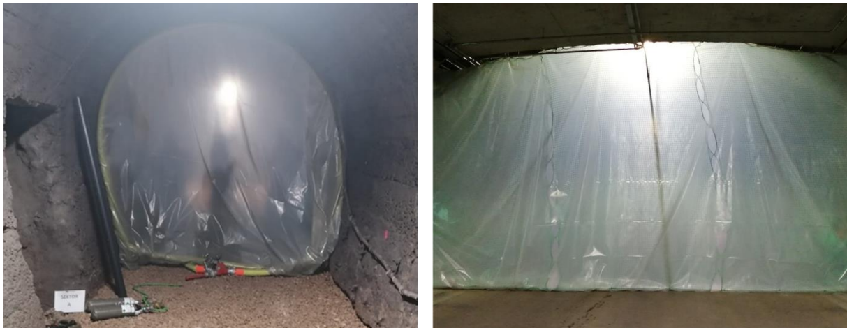
Figure 2: Left: The hose brattice - "Scheuer model" - a very easy and quick to erect option for small cross-sections (Photo: ÖBH, Scheuer). Right: Initial prototype of the mobile ventilation door made of plastic film and nets (Photo: Hofer).
